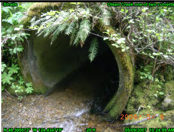
Image-829: Olsen Creek one of two culverts
